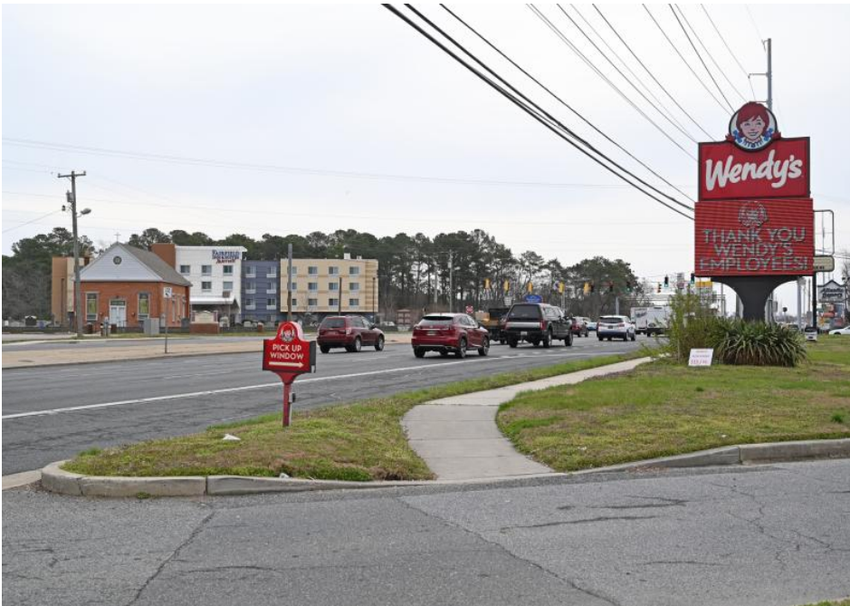
A project is planned to lengthen the turn lane on southbound Route 1 at Old Landing Road and eliminate one of the two turn lanes on northbound Route 1 into the Rehoboth Mall shopping center. The goal is to begin construction this spring. NICK ROTH PHOTO
