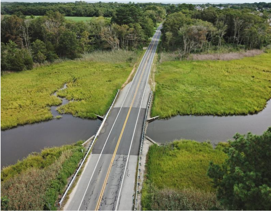
The New Road bridge over Canary Creek in Lewes is set to be replaced. Roadway construction will begin fall 2024 with completion in 2025. NICK ROTH PHOTO
