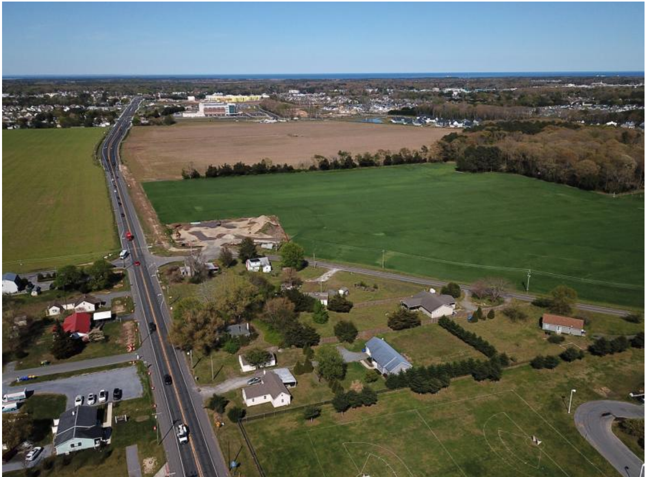
The second phase to widen Route 24 from Mulberry Knoll Road to Love Creek is expected to begin construction this spring. A traffic signal will be installed at the intersection of Route 24 and Mulberry Knoll Road early in the process. NICK ROTH PHOTO
