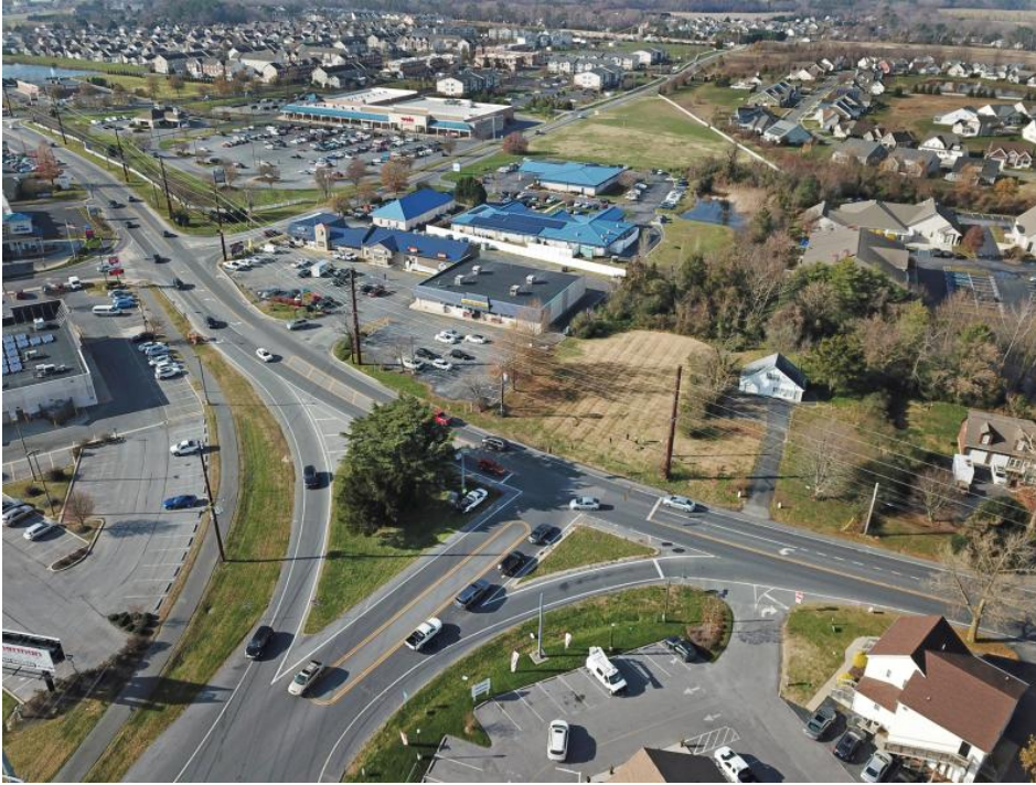
Old Orchard Road will be aligned with Wescoats Road at the existing traffic signal on Savannah Road. Construction is set to begin in fall 2024. NICK ROTH PHOTO
